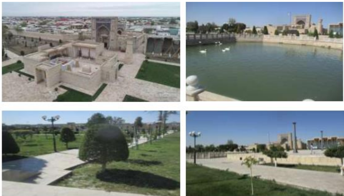
Figure 2. The condition of the Abdukholiq Gijduvani complex after 2018.
