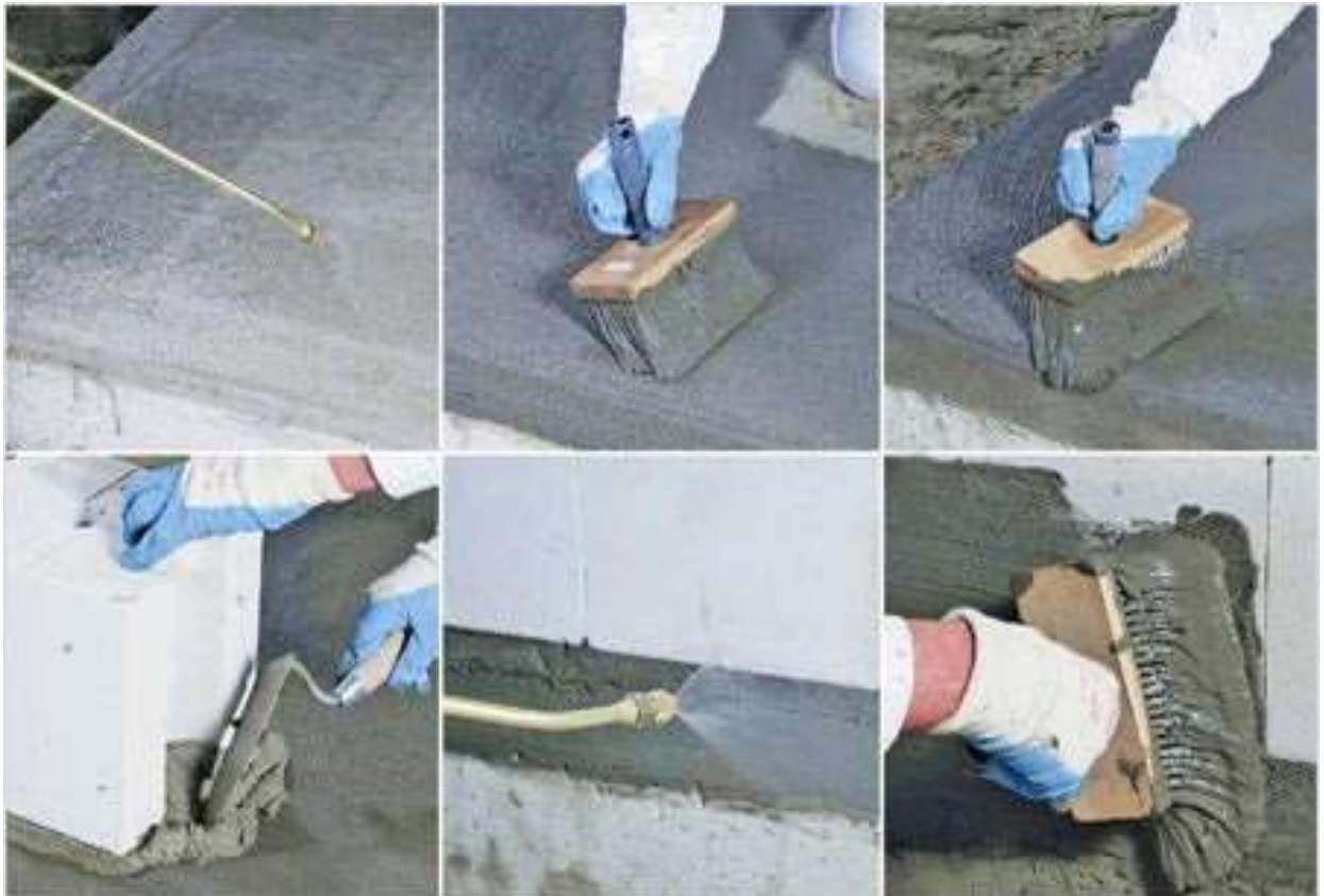
Fig. 1 Methods for applying Penetron waterproofing material to various surfaces
